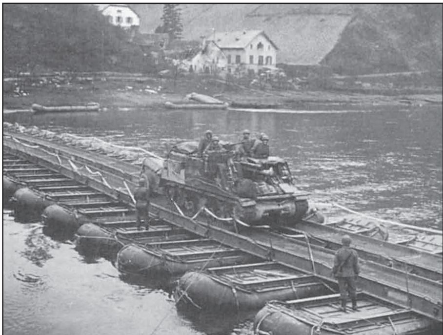
Typical pontoon bridge
