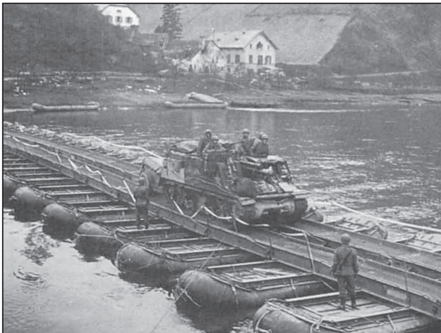
Typical pontoon bridge
